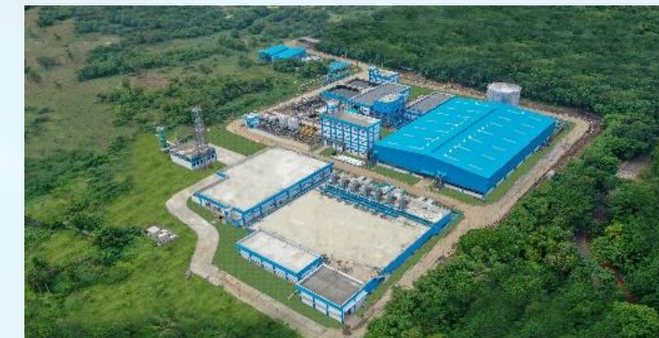
45 MLD Koyambedu TTRO Recycle Reuse Plant, Chennai, India One of the largest and technologically most advanced water reuse plants in India ensuring Chennai's Water security
