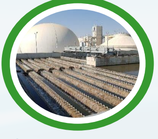
Sludge Treatment & Energy Recovery
