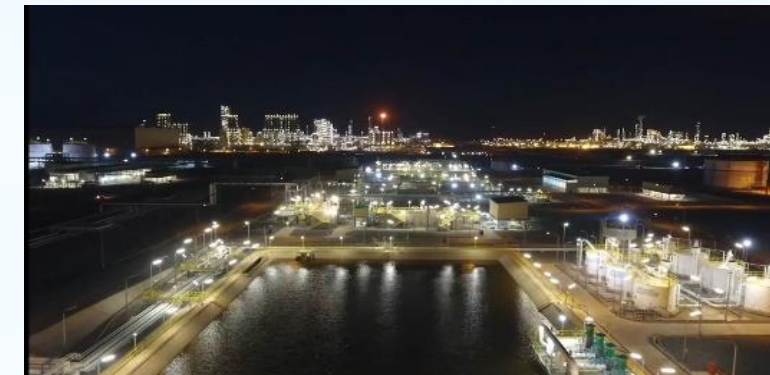
102 MLD Industrial Effluent Treatment Plant for PETRONAS, Malaysia Largest industrial Effluent Treatment Plant in South East Asia
