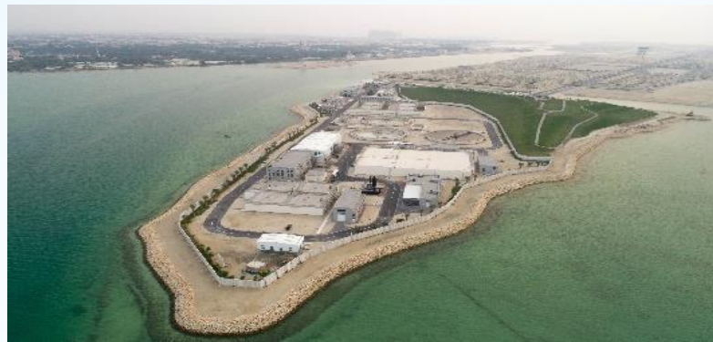
Al Madina Al Shamaliya 40 MLD Sewage Treatment Plant, Bahrain Awarded Wastewater Project of the Year at Global Water Awards, 2019
