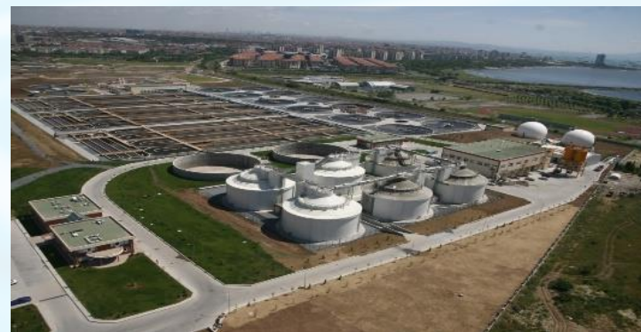
Total City Water Management, Istanbul, Turkey Managed 124 units catering to 16 million population in the Asian and European districts of Istanbul
