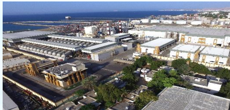
191 MLD SWRO (Desalination) Plant, Al Gubrah, Oman Largest desalination plant in the country of Oman
