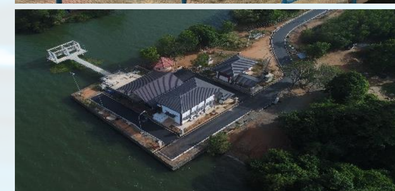
32 MLD Drinking Water Treatment Plant, Dambulla, Srilanka Integrated water supply scheme with transmission, distribution and water treatment
