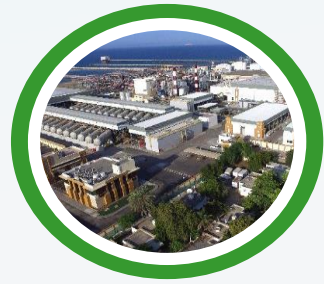
Sea & Brackish Water Desalination
