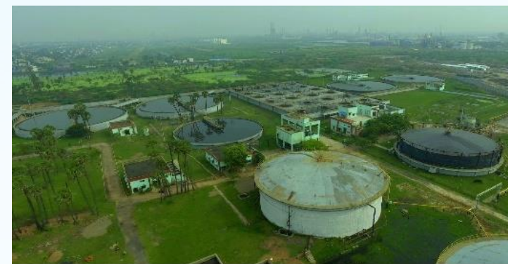
110 MLD Sewage Treatment Plant, Kodungaiyur, Chennai, India One of the most energy efficient and energy neutral STPs in the country
